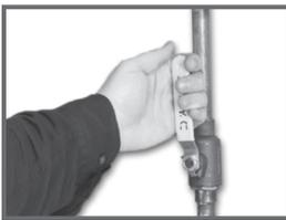
1. Confirm the inlet ball valve to the system is off, then turn on the main supply line to the system.
